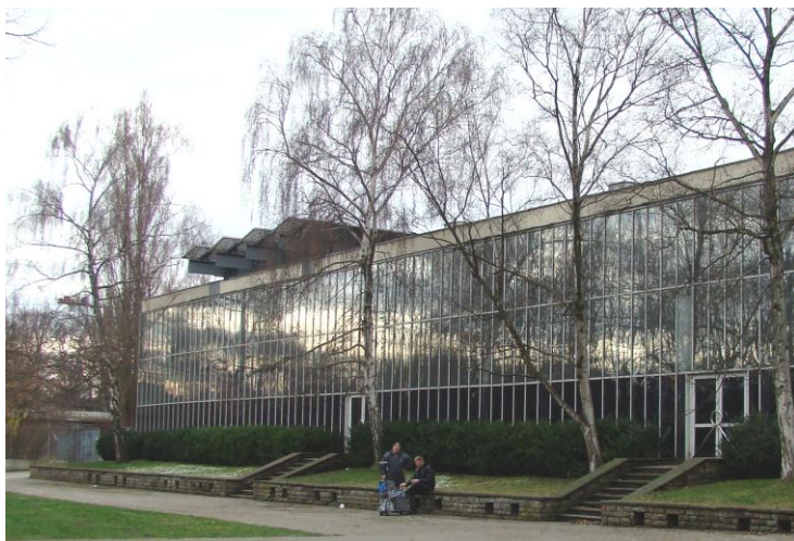
Mobile measurement set up in front of Glashalle
